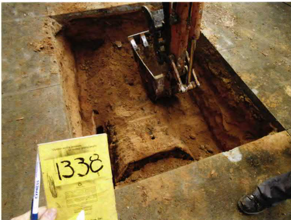
Picture 1: UST 1338Albatross during excavation.
