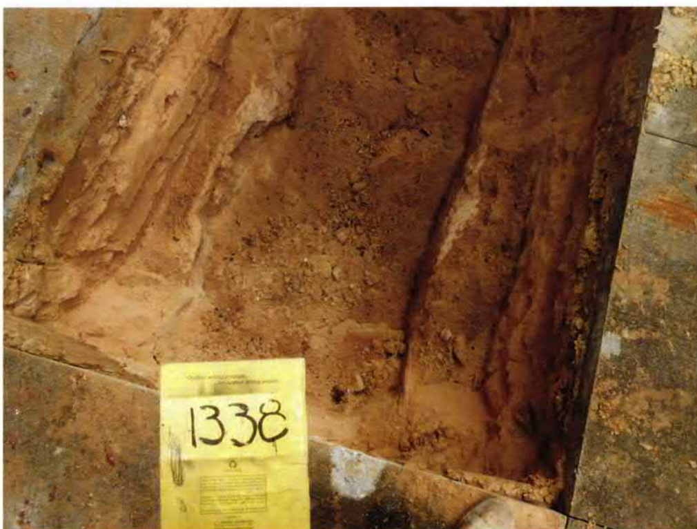
Picture 2: UST 1338Albatross excavation.
